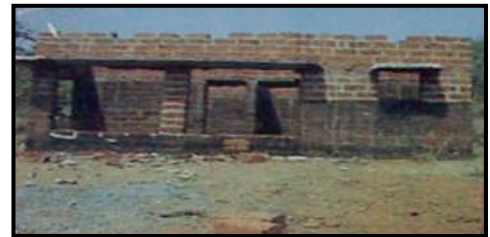
Photo of incomplete Mahavir Community Hall at Tadaki Hill side, Khordha
